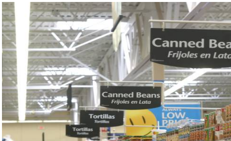
Store lights dim based on available daylight
